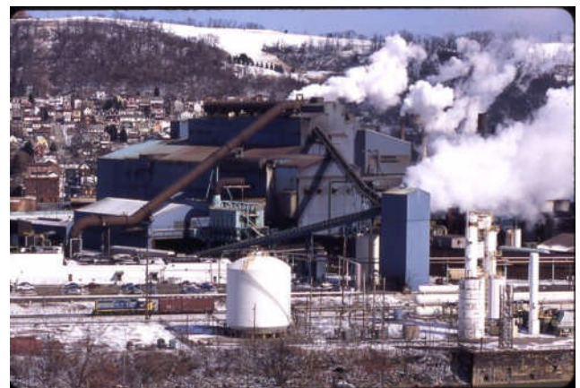
CSX local L121 is dwarfed by the massive USS Edgar Thomson foundry
